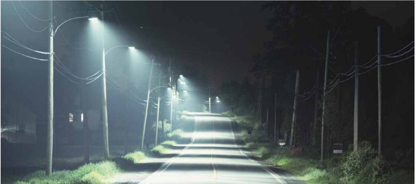
Discomfort and disability from intense, blue-rich LED lighting can decrease visual acuity and safety, creating a road hazard.
