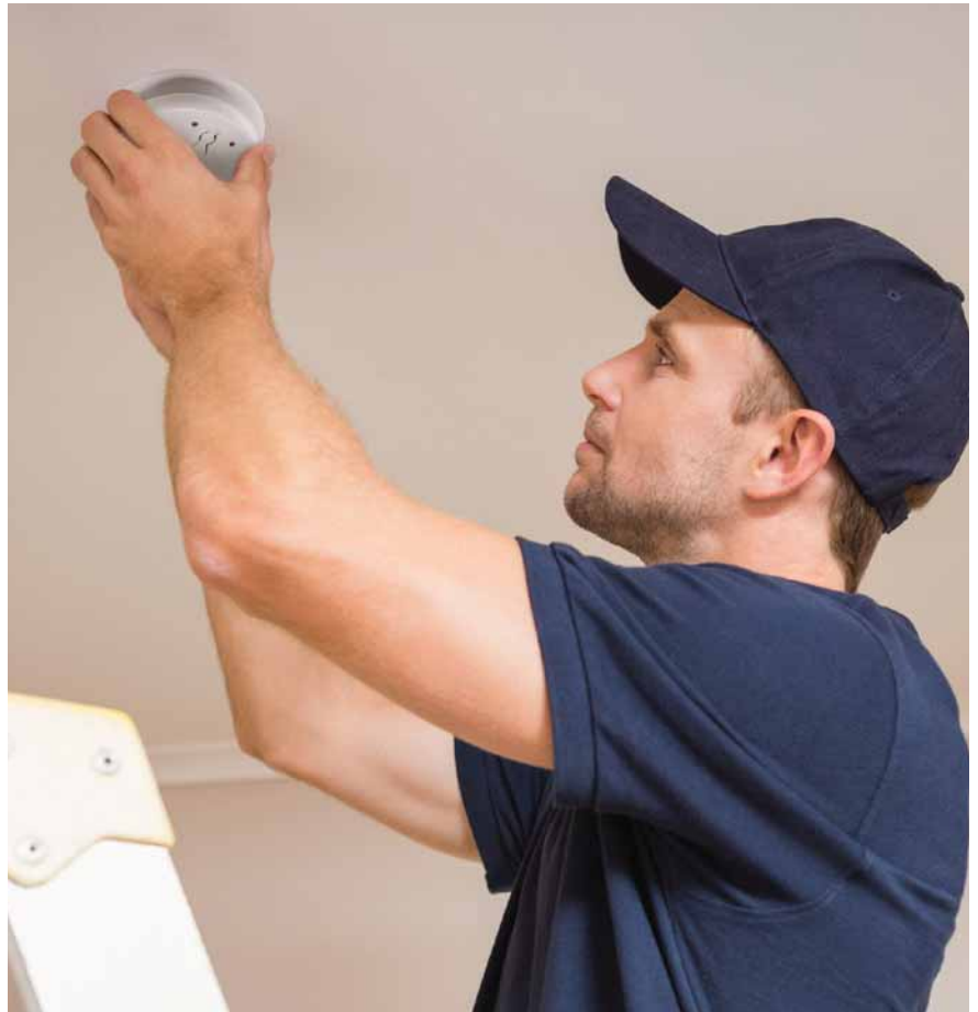
The heat is on for ionisation alarms as units fail to activate in the event of a fire.
