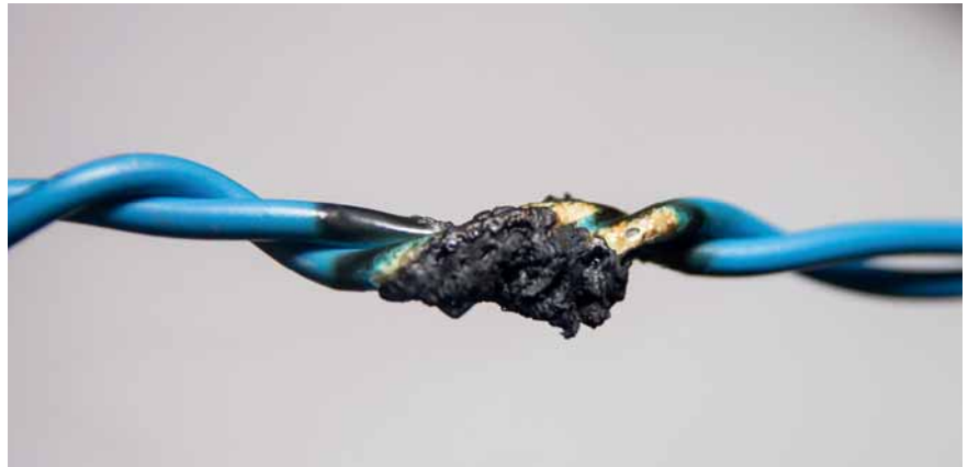
Heat rise in cabling could cause fire or cable failure
