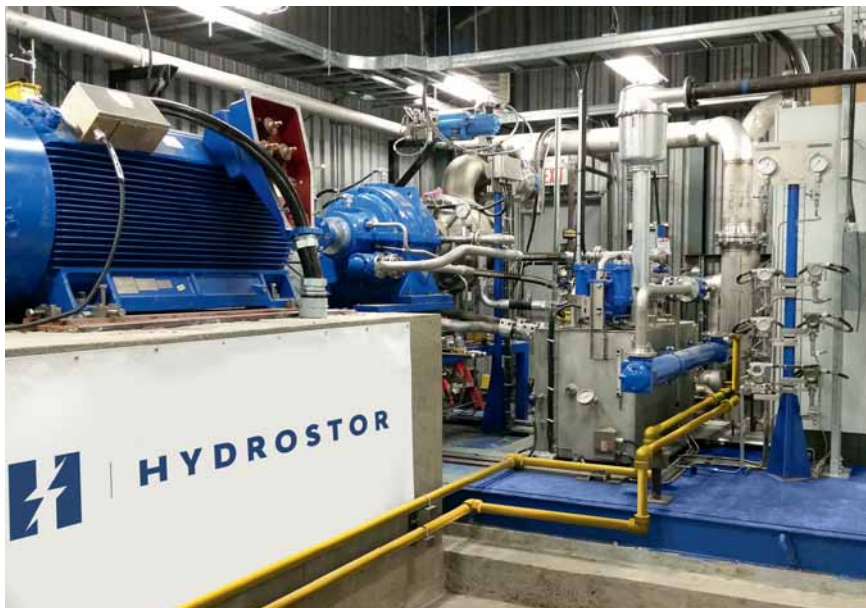
Demonstration prototype of Hydrostor's A-CAES compressed air storage system in Toronto, Canada.
