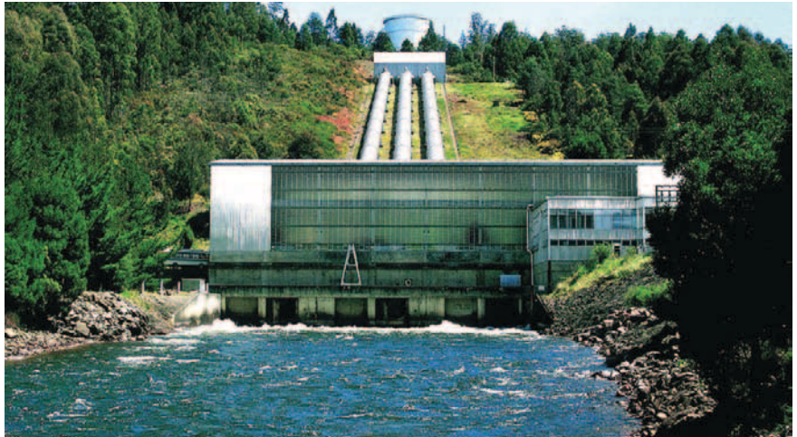
The Liapootah Power Station was commissioned in 1960 and is one of 11 hydro-electric power stations that make up the Derwent scheme.
