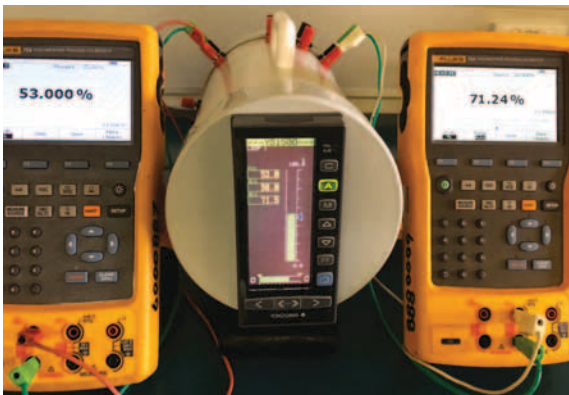
Proportional band set to 100% therefore a controller gain of one. Integral time set to 10 seconds therefore six repeats per minute. 3% error on input results in a 3% change of output followed by 18% output ramp over one minute.
