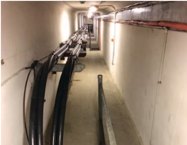
The narrow high voltage cable tunnel was only 1.6m wide.
