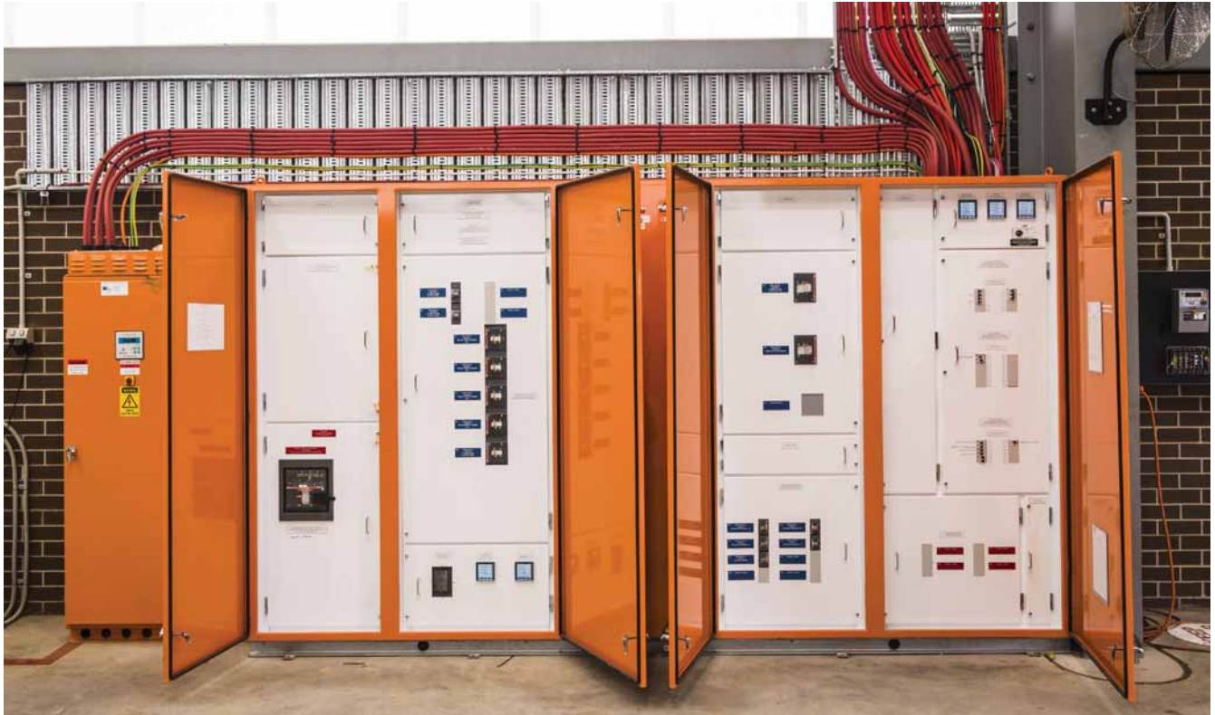
Several of the electrical services needed to be installed in the ground at least two months before the building was erected.
