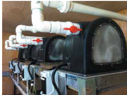
PowerSpout generators piggy backed to make the most of the available water.
