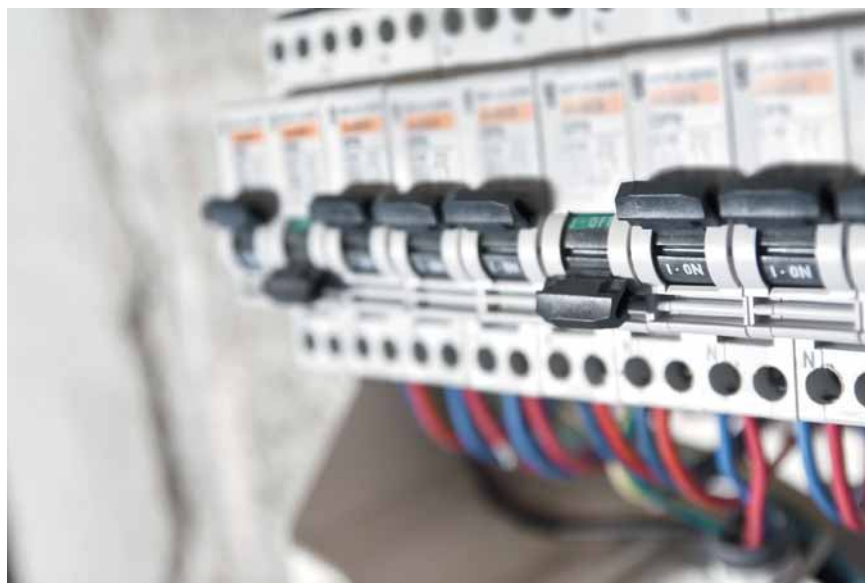
This residual current device interrupts both conductors.
